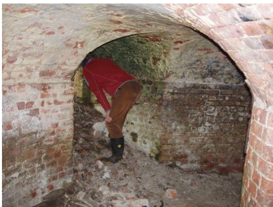
Inside a disused Norfolk limekiln, showing vaulted, brick-built construction and central column with extraction chute descending from the firing pot above.
