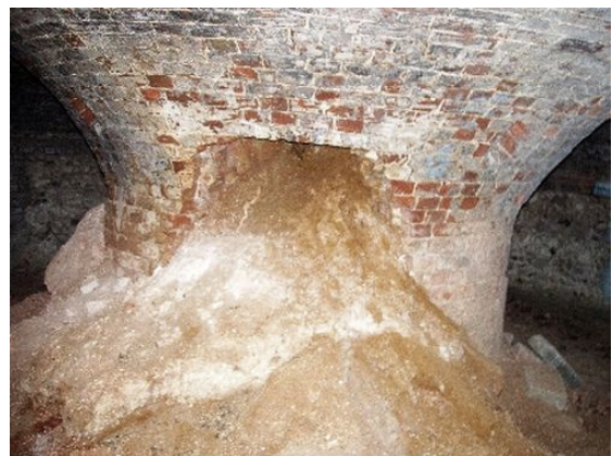
Inside a disused Norfolk limekiln, showing vaulted, brick-built construction and central column with extraction chute descending from the firing pot above.
